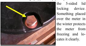
The 5-sided nut is turned counterclockwise to remove the lid.
