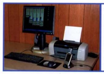
This equipment is part of the SCADA telemetry operating from the District Office. The graphs feature the new elevated tank, Novinger, Pure Air, and Clay booster pump stations and shows which pumps are running and tank levels among other important information regarding daily operations.
