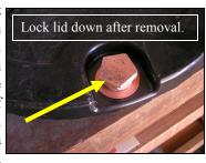
a 1" socket, a vice-grip type or slip-joint pliers can turn the 5-sided lid locking device. Something placed over the meter in the winter protects the meter from freezing and locates it clearly. A simple electric fence post might be used if you don't place protection over the pit in cold weather.
