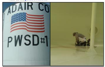
Yes, you see a painter inside a tank. He has sandblasted the tank, removed all rust and other foreign materials, and is putting the finishing touches on an epoxy coating to make the water safe and clean for your use when the tank is refilled.
